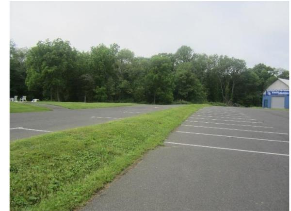
Multiple rows of parking spots in the parking lots can be replaced with porous asphalt to capture and infiltrate stormwater. A preliminary soil assessment suggests that more soil testing would be required before determining the soil's suitability for green infrastructure.
