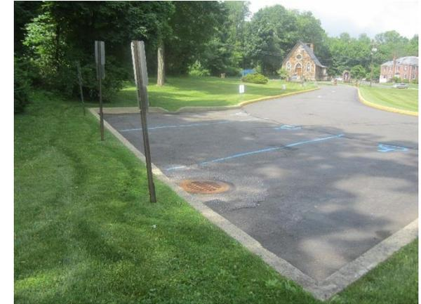
Multiple rows of parking spots can be replaced with pervious pavement to provide stormwater an opportunity to infiltrate. Building a rain garden adjacent to the northwest corner of the church can capture, treat, and infiltrate roof runoff. A preliminary soil assessment suggests that the soils have suitable drainage characteristics for green infrastructure.
