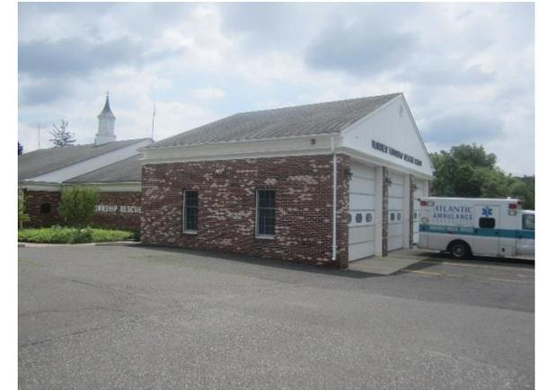
Parking spots around the complex can be replaced with porous asphalt to capture and infiltrate stormwater. A preliminary soil assessment suggests that the soils have suitable drainage characteristics for green infrastructure.
