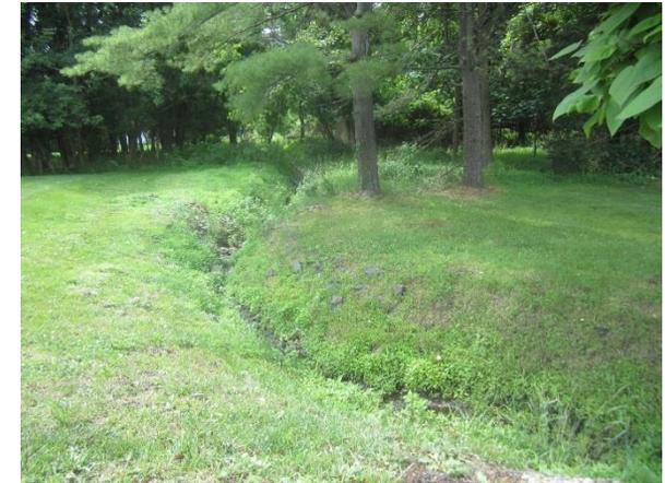
Stormwater is currently directed to an existing trench. Parking spots west and south of the building can be replaced with porous asphalt to capture and infiltrate stormwater. A preliminary soil assessment suggests that more soil testing would be required before determining the soil's suitability for green infrastructure.
