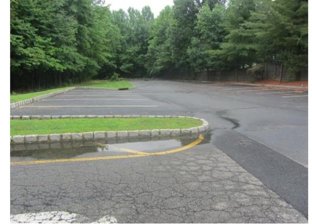
Two rows of parking spots south of the school can be replaced with porous asphalt to capture and infiltrate stormwater. A preliminary soil assessment suggests that more soil testing would be required before determining the soil's suitability for green infrastructure.
